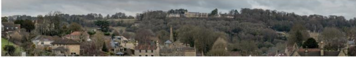
PROPOSED, ZOOMED IN: Photomontage View from The Tyning Road, Freshford looking towards the site - planting shown as year 1
