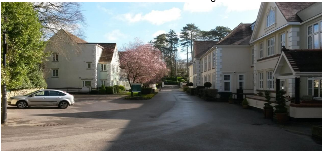
On site view looking east – with Hillcrest House/ Fountain Place to left and Alexander Heights to the right (both 2.5 storey buildings with rooms in the roof space both identified for demolition).
